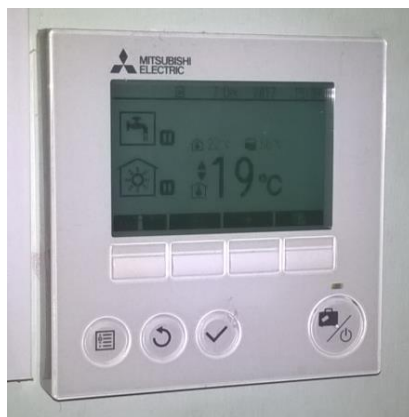
Figure 2.16 ASHP heating and hot water system controller (above) and manual (left)
