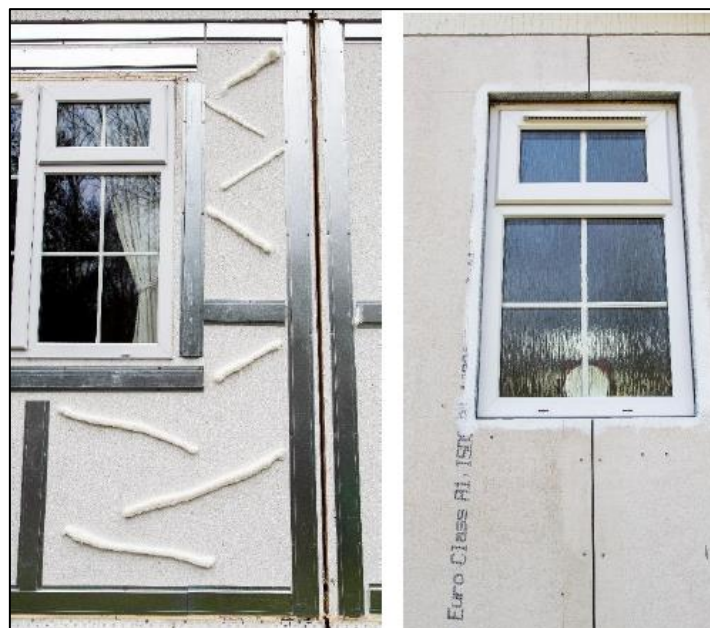
Figure 3.4a Top-hat rails and Instafoam on park home 20
