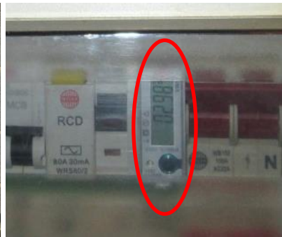
Figure 3.2 – Pictures of SIG solar sharer technology installed (a) inverters in loft space (b) SES in fuse box
