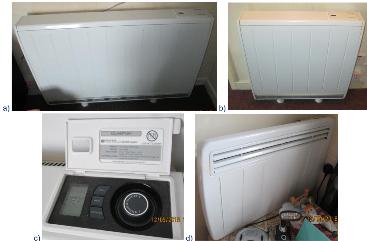
Figure 3.1 Example of the Dimplex Quantum storage heaters installed in homes in this study (a) large (living room) (b) smaller (hall) (c) close up of controls (d) panel heater fitted in bedroom 2 of 2-bed flats
