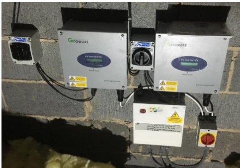
Figure 3.2 – Pictures of SIG solar sharer technology installed (a) inverters in loft space (b) SES in fuse box
