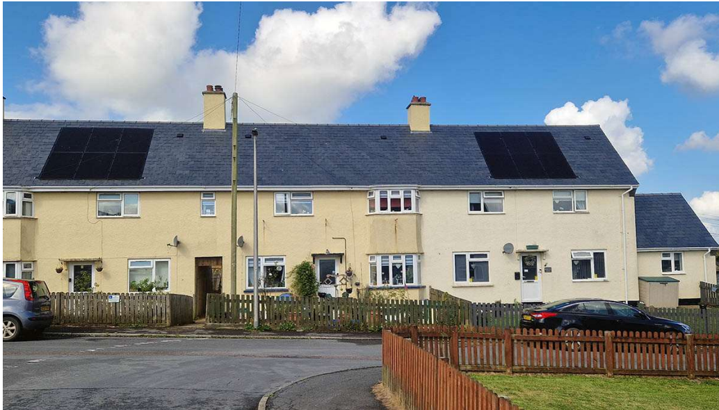
Figure 2.3 Two houses with east-west facing in-roof solar PV installations
