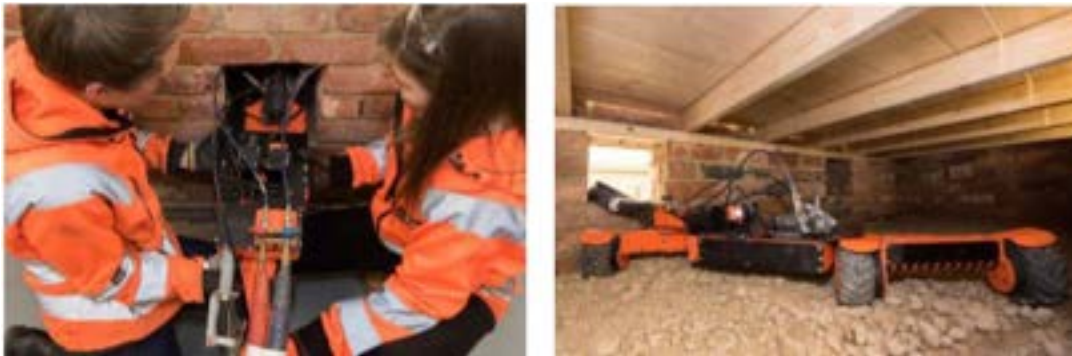
Figure 3.1 (b) Q-Bot being inserted into the under-floor space
