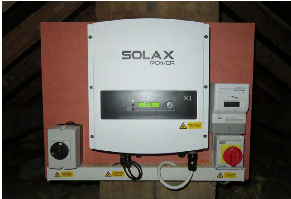
Figure 5.3 SolaX inverter with the DC isolator, AC isolator and smart generation meter
