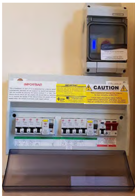
Figure 7.3 AC isolator and generation meter in an enclosure above the consumer unit
