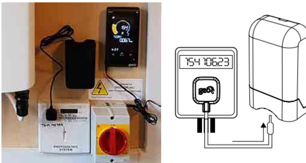
Figure 2.2 (a) GEO Solo PV II installation (b) Schematic showing LED sensor and transmitter
