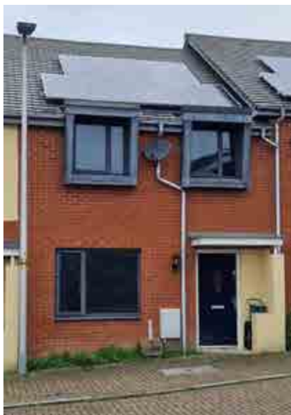
Figure 4.27 Property with 1.75kW solar PV system
