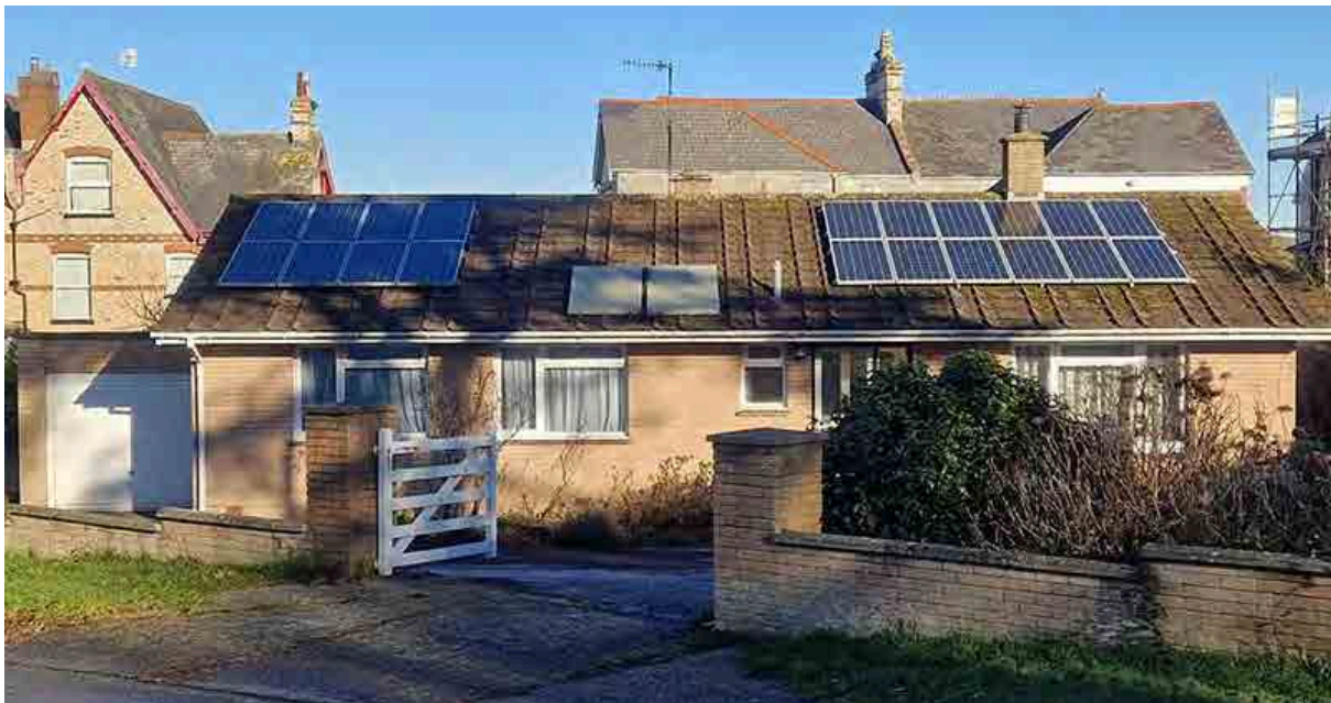
Figure 4.2 Household W-01 with solar PV arrays on the left and right and 2 flat-pate solar thermal collectors in the middle of the roof
