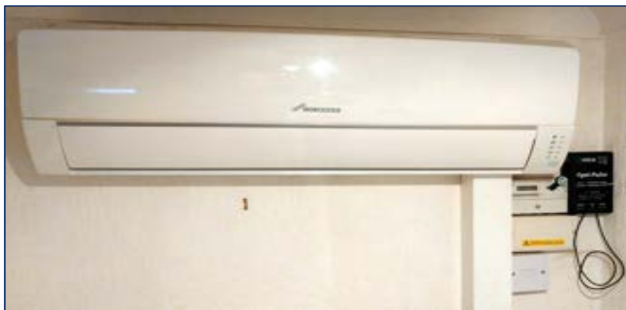
Figure 2.6 Indoor unit of ASHP with watt hour meter and Optipulse sensor
