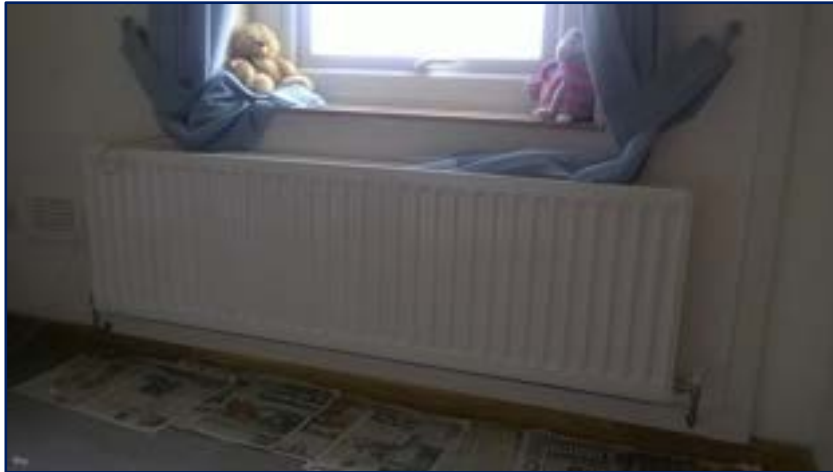
Figure 3.3 Oversized radiators
