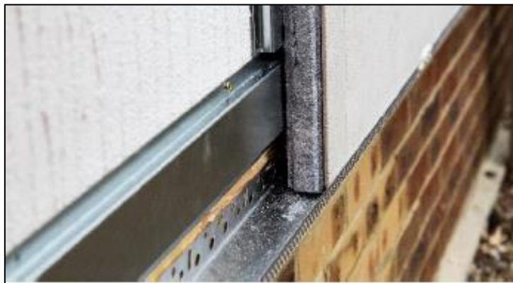
Figure 3.3 InstaClad panel slotting into the starting rail on an EWI installation 20
