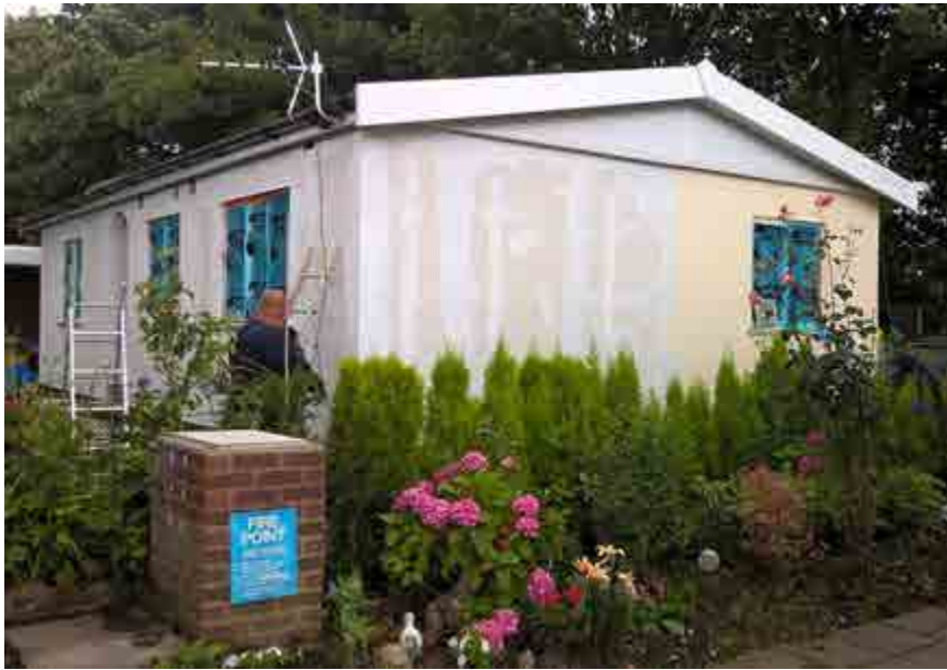
Figure 3.5 Park home retrofit showing joint filler on the InstaClad panels (left) and the final rendered surface (right)
