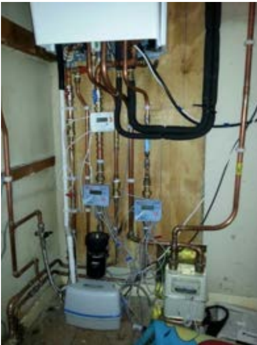
Figure 3.11 picture of pipework, and monitoring equipment below a boiler / hydrobox, showing gas meter and 3 heat meters.
