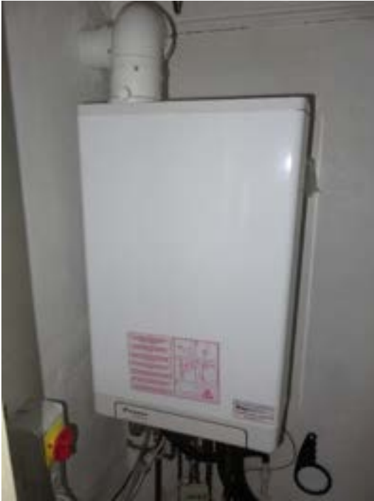
Figure 3.4 Boiler / hydrobox installed in an airing cupboard
