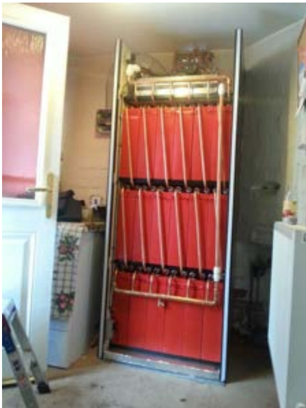
Figure 3.7 Sunamp heat battery with the cover removed showing the cells of PCM and plate heat exchanger at the top.
