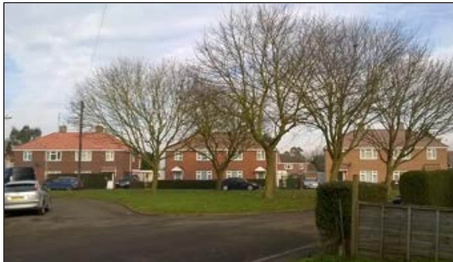
Figure 2.1 Example of a property receiving a smart thermostat installation
