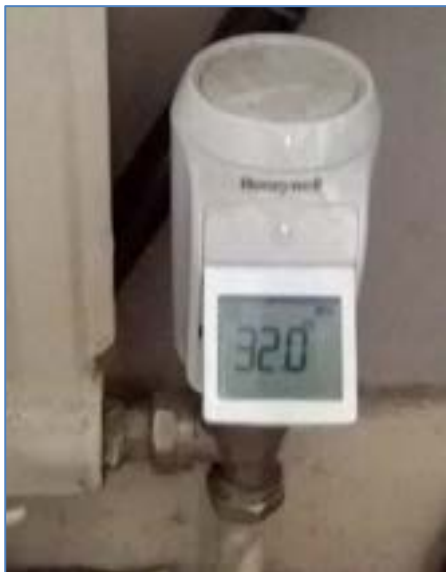
Figure 2.7 Honeywell HR92 smart TRV
