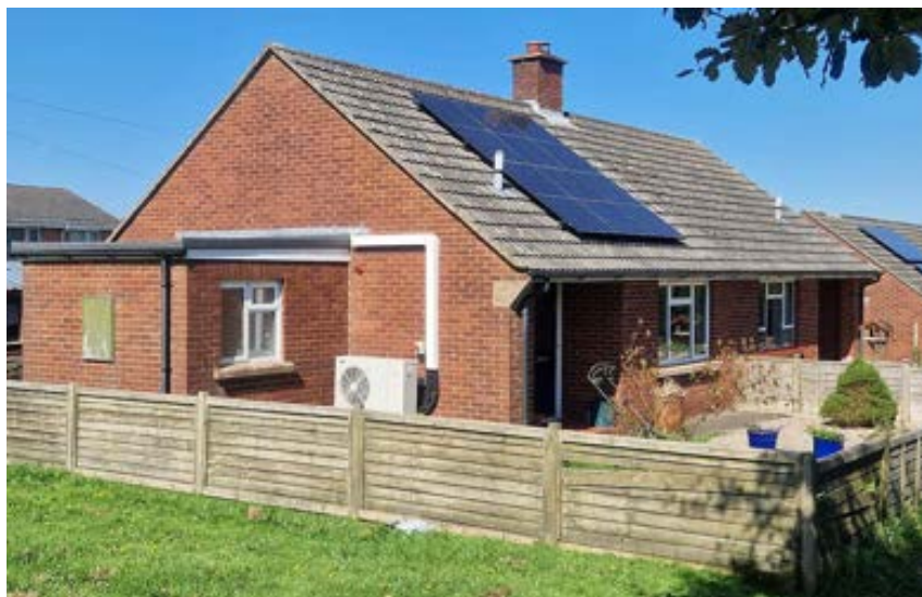
Figure 2.2 Semi-detached bungalow with solar PV, ASHP and a Mixergy cylinder
