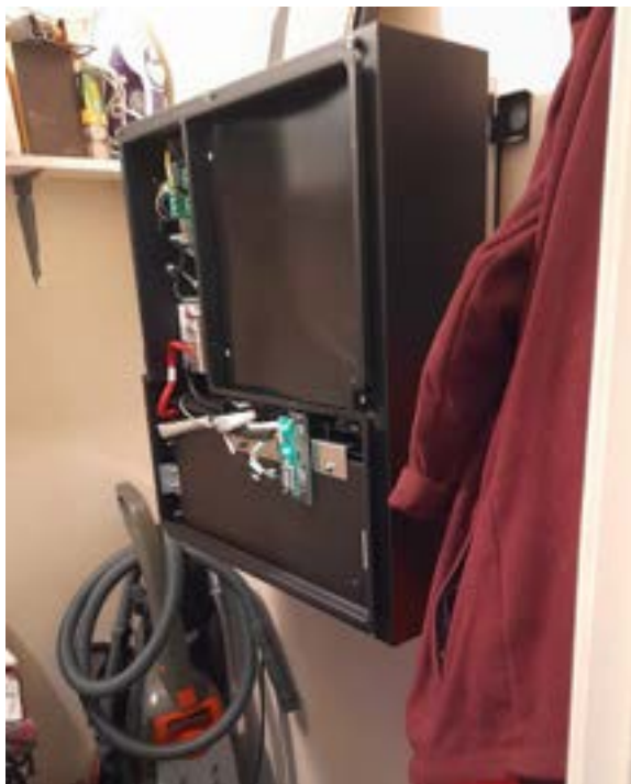
Figure 3.17 Alpha ESS SMILE-B3 battery with the cover off
