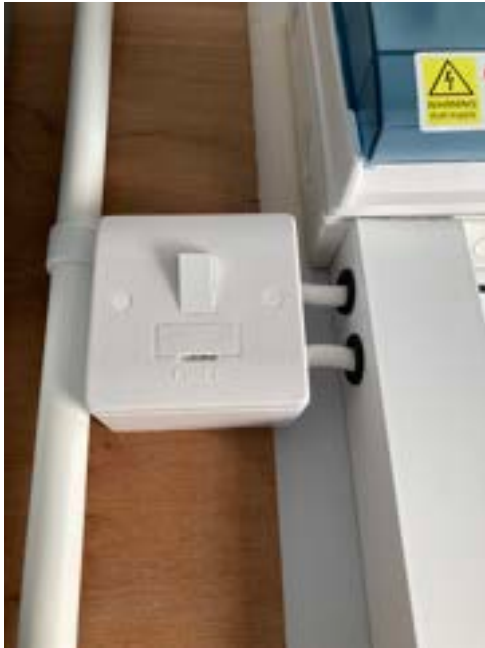
Figure 3.3(a) Isolator installed by engineer Figure 3.3(b) SMILE-B3 battery breaker and switch
