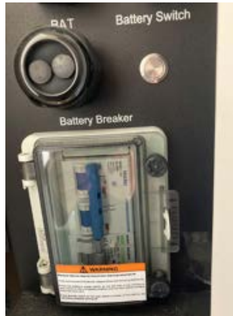
Figure 3.3(a) Isolator installed by engineer Figure 3.3(b) SMILE-B3 battery breaker and switch
