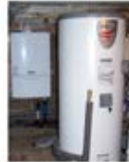
This is a standard gas boiler. You will have a separate boiler and hot water tank.
